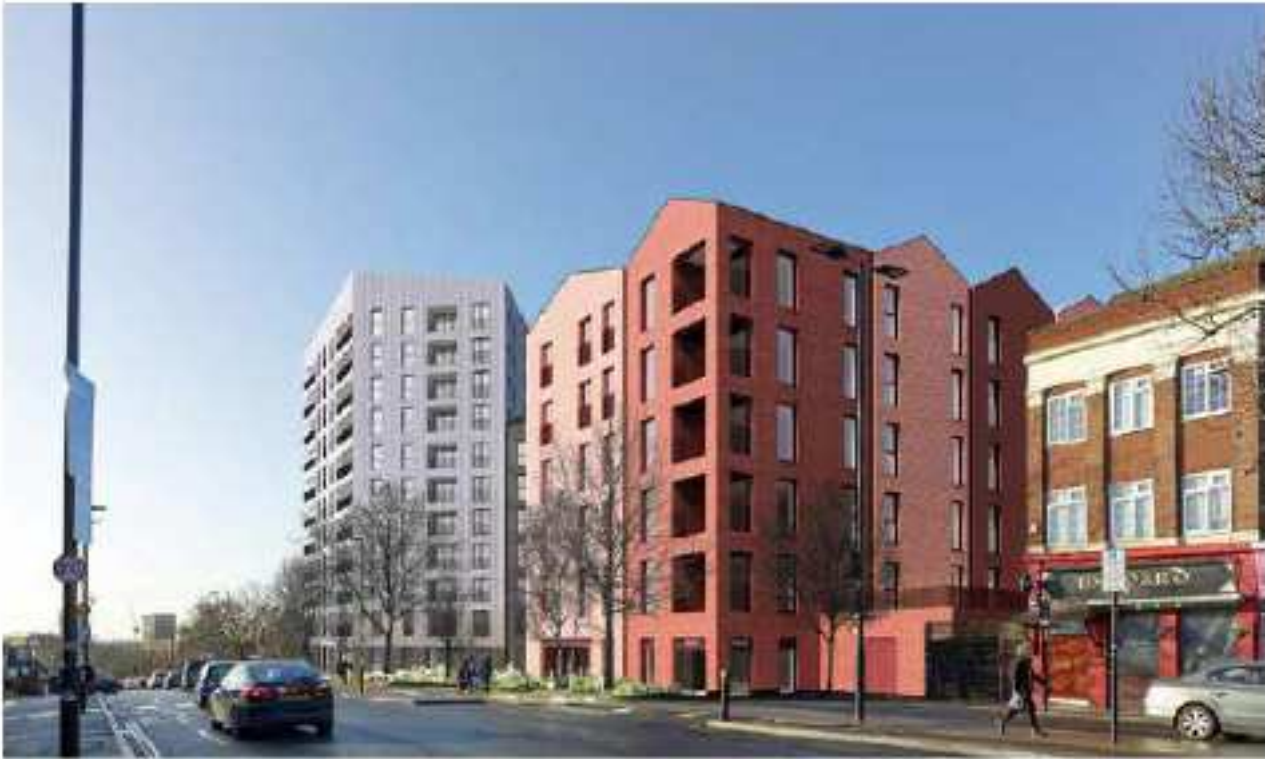
View of Proposed Development from Greenford Road (from north)
